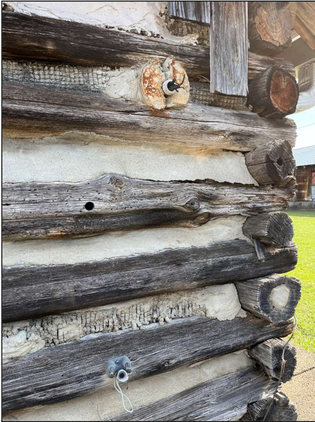
Degraded chinking and daubing West Elevation
