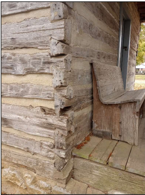
North Elevation: Rotted Logs
