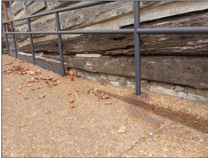
Northwest Elevation: Chinking and Daubing Damage
