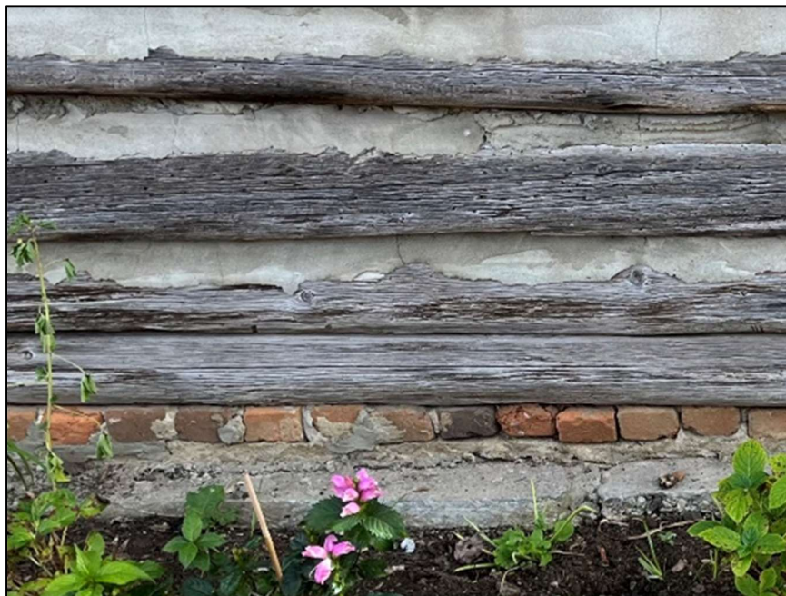
Brick Foundation with Missing Mortar West Elevation
