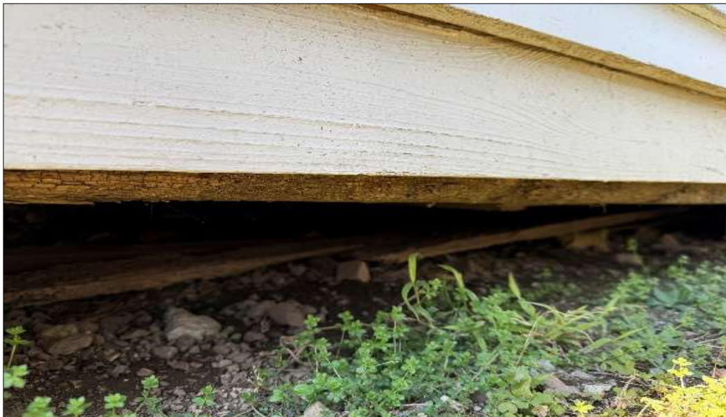
Lack of Moisture Barrier Beneath Structure
