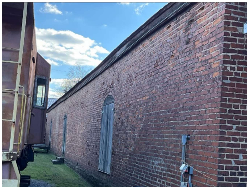
East Elevation Roof (No Gutter)
