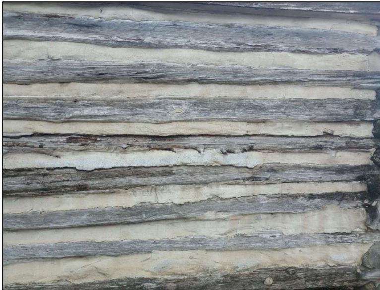
West Elevation: Chinking and Daubing Damage
