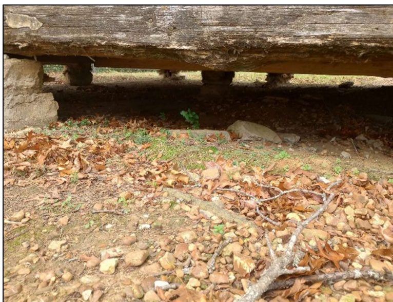
East Elevation: Drainage Issue Under Building
