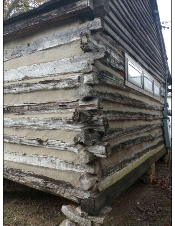
Northwest Elevation: Rotted Logs
