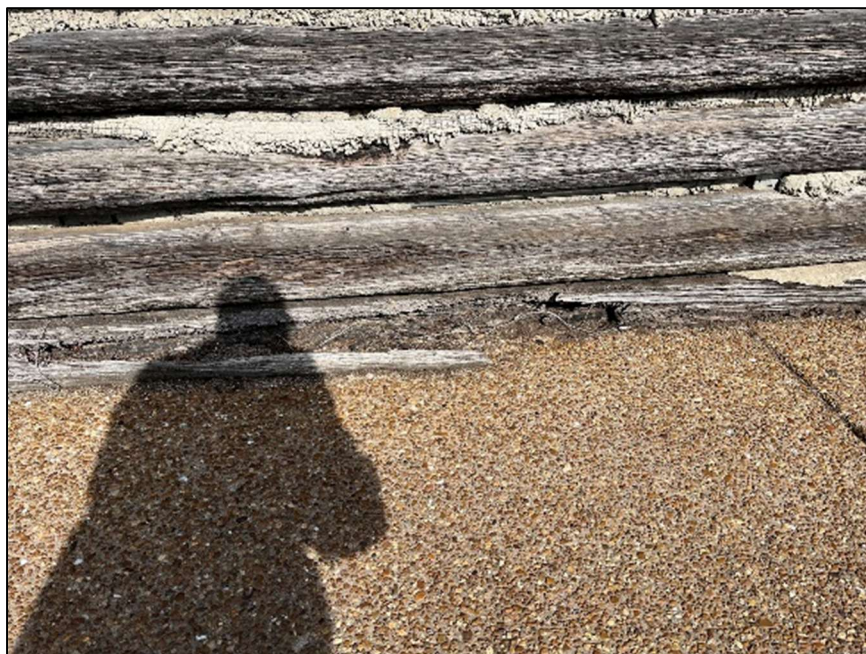
Degraded Logs South Elevation
