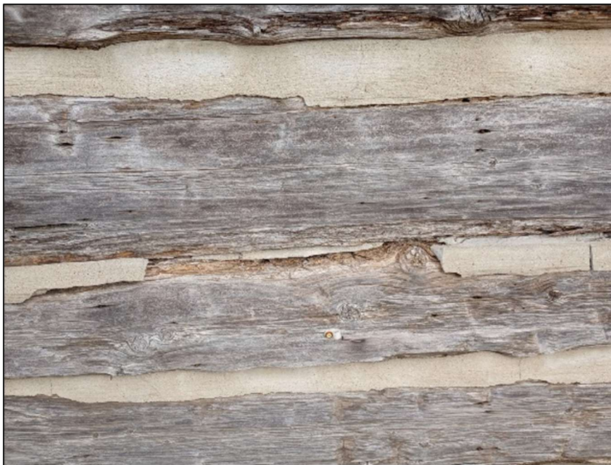
Chinking and Daubing Damage
