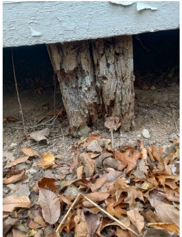
Damaged Wood Foundation Block
