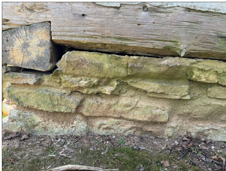
Gaps Between Wood and Foundation West Elevation
