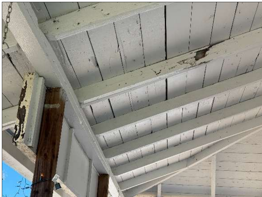
Rotted Beams for Front Porch Roof
