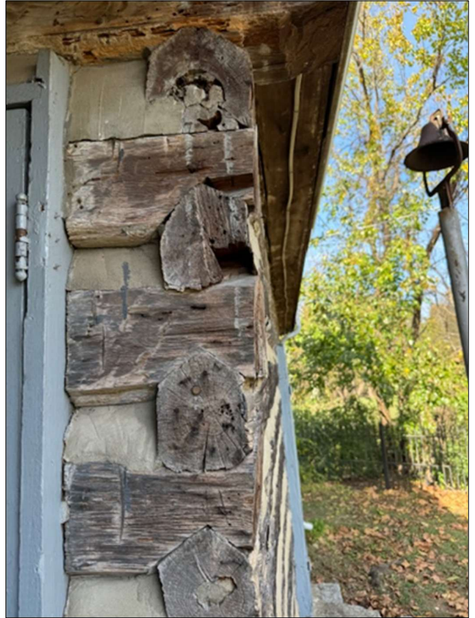
Half Dovetail Notching with Holes Southeast Elevation
