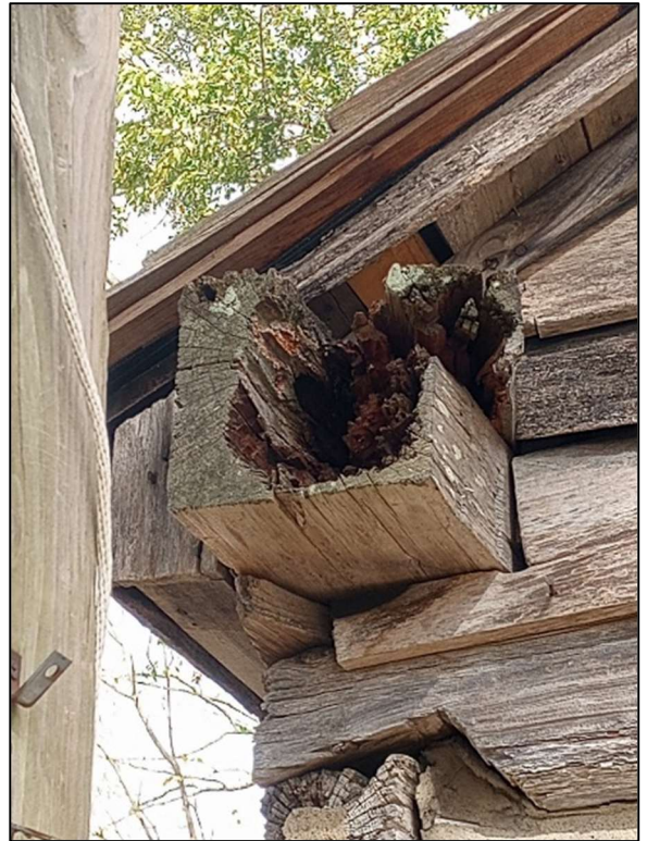
Southwest Elevation: Rotted Logs
