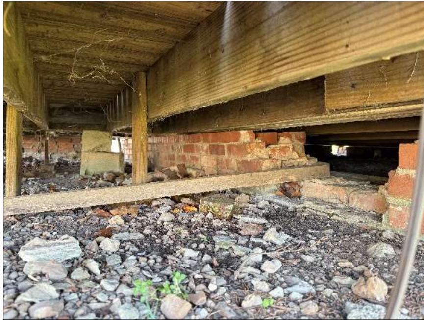
Lack of Moisture Barrier Beneath General Store
