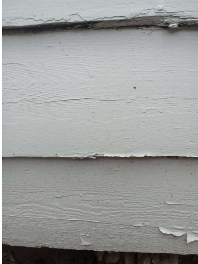
West Elevation: Peeling and Chipping Paint
