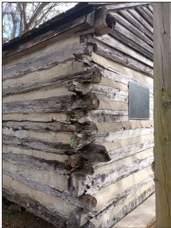
Southwest Elevation: Rotted Logs
