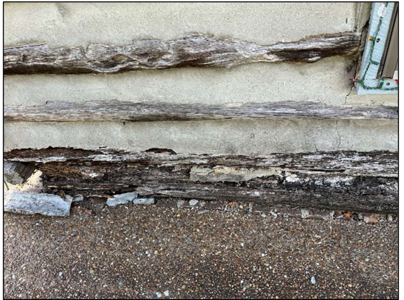
Degraded logs North Elevation
